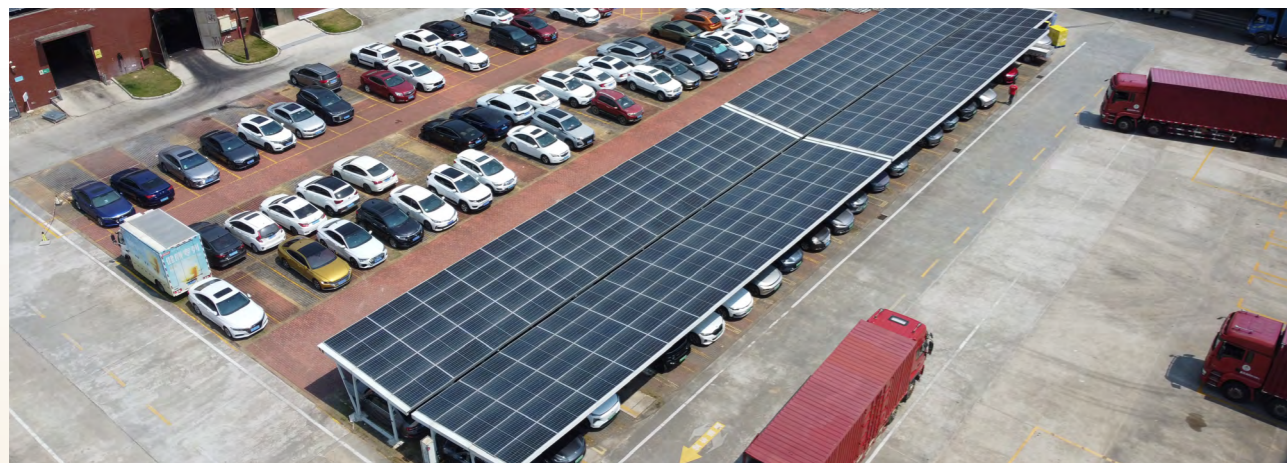
Photovoltaic (PV) Carport
